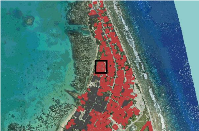
Figure 10: Location of Princess Margaret Hospital, Funafuti and Buildings currently impacted by climate change hazard damage. The red highlights buildings that are exposed to hazards present day. (Source: Tuvalu Coastal Adaptation Project.)
