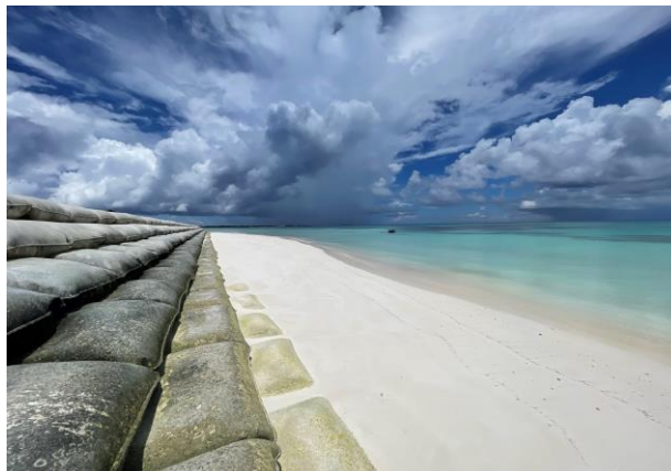
Seawall in Tuvalu. (Source: Tuvalu NAP Project-Mission 2024.)
