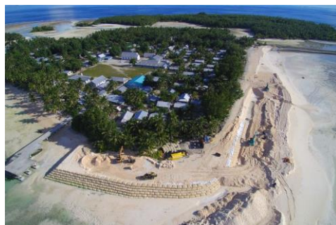
Rebuild of seawall in Nukufetau. (Source: CSIRO, Federation University, Climate Comms (2024))
