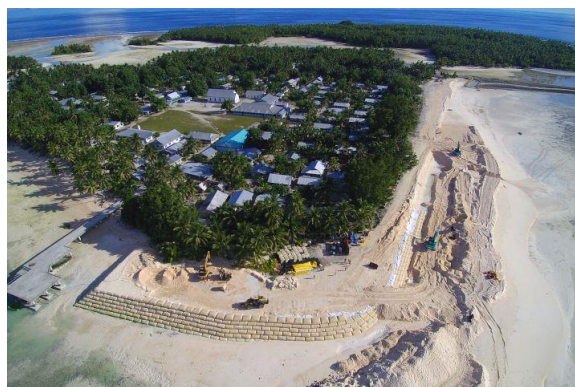
Figure 9-13: Borrow pit filling project at Funafuti (Source: [35])
